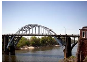
Edmund Pettus Bridge Selma, AL
